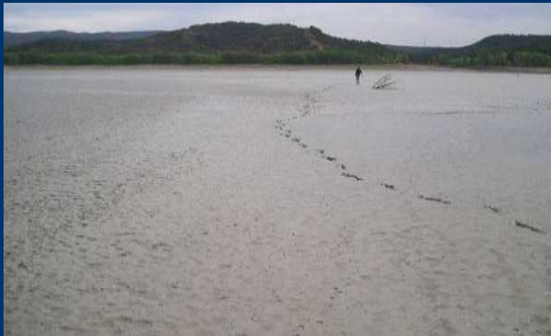
Deposition of suspended sediments in the Barasona reservoir, Èsera River, Spain
