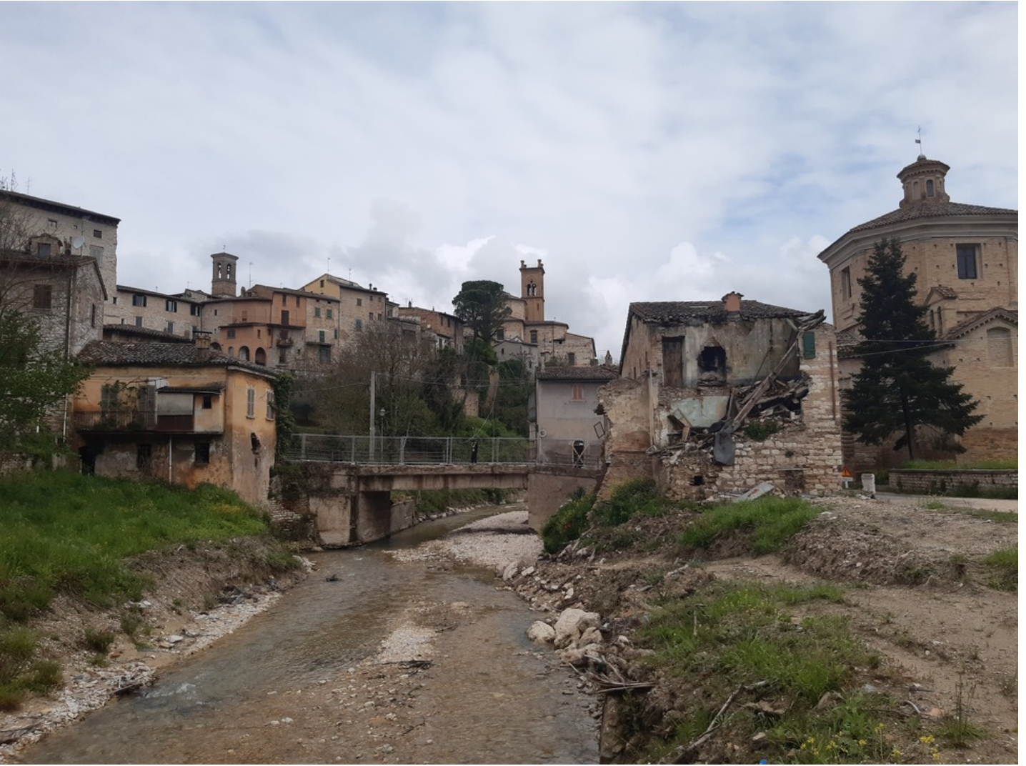
Figure 11: In Pergola damages occurred only below the ancient city walls. Houses which were built close to the river and the (clogged) bridge were heavily damaged.
