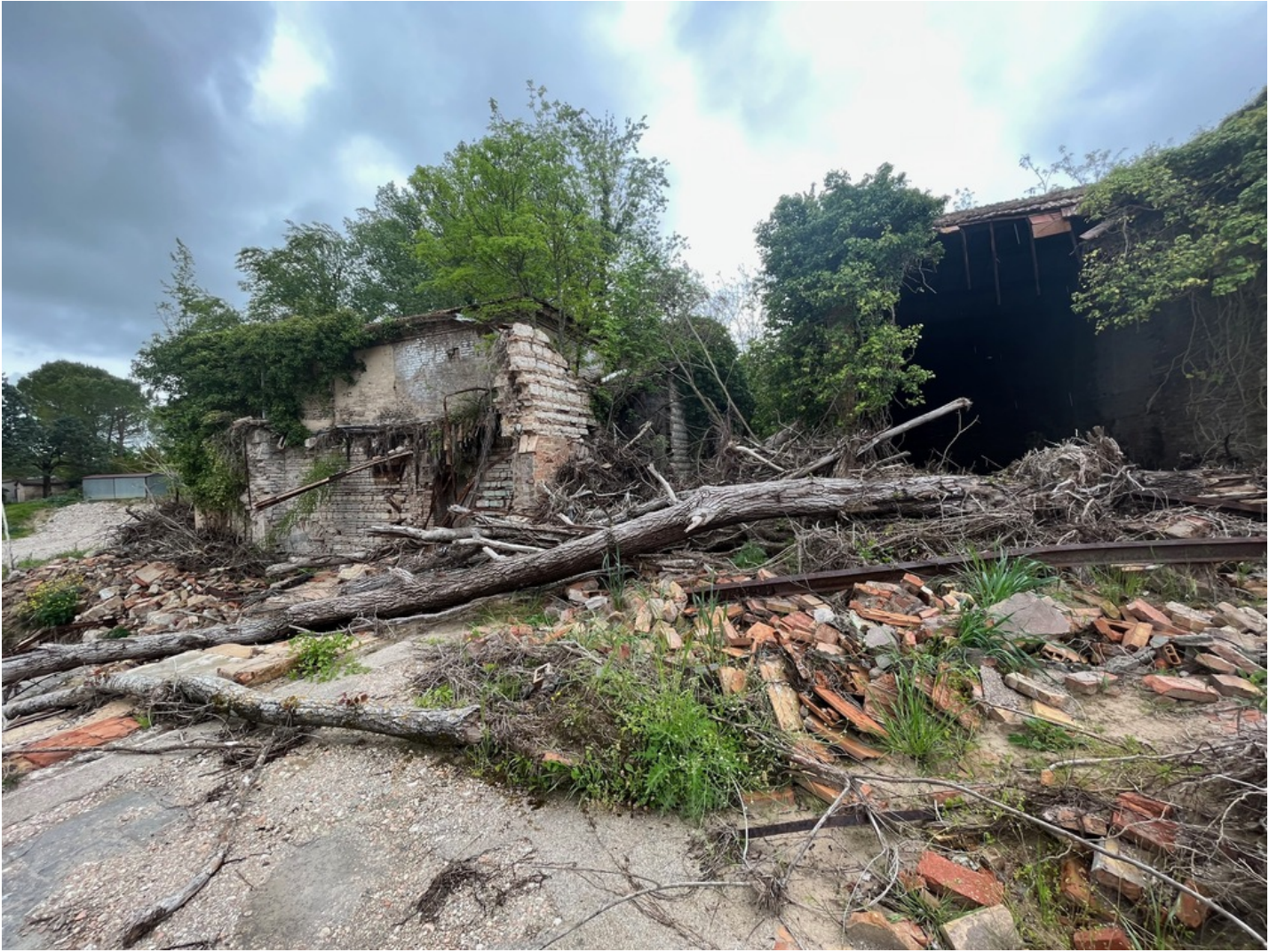
Figure 8: Uprooted trees causing damages.
