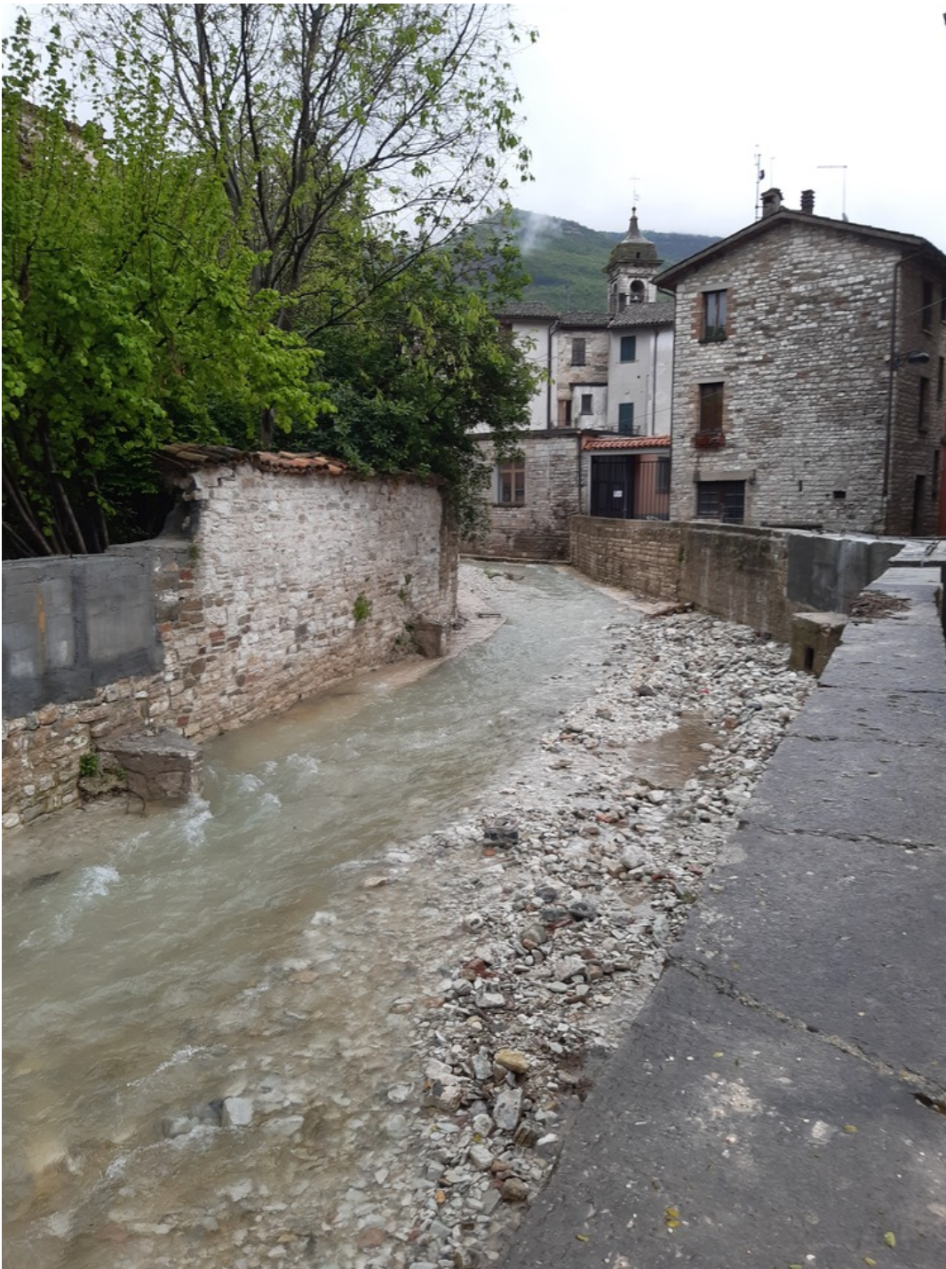
Figure 10: Artificial channel in the city of Cantiano. Spilling over of these channels flooded the whole city center.
