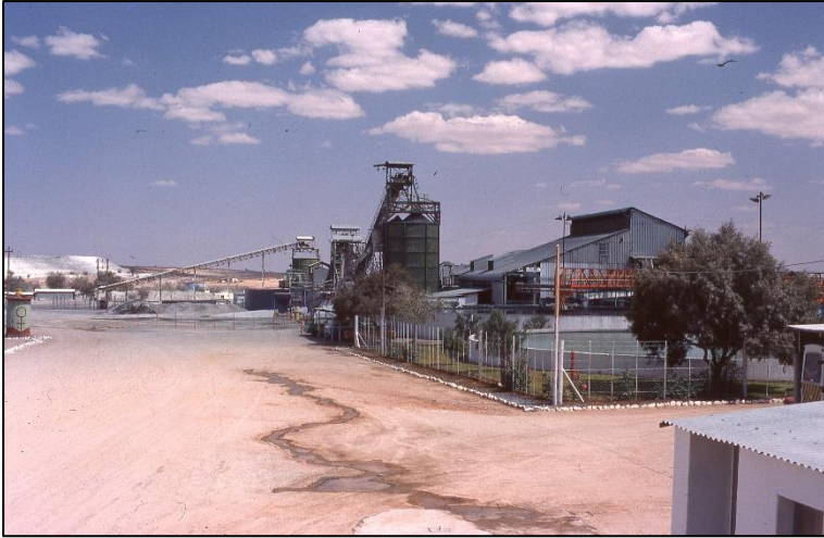
Van Zyl Shaft and plant ca. 1984 (Photo: G Borg)
