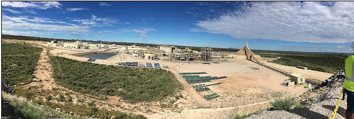
The Otjikoto Gold Mine Plant (Photo: G Schneider)
