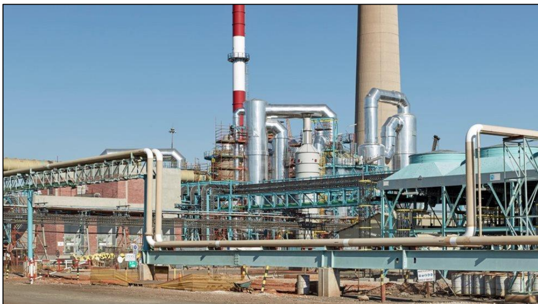
The acid plant, part of the Tsumeb smelter ( www.metso.com )
