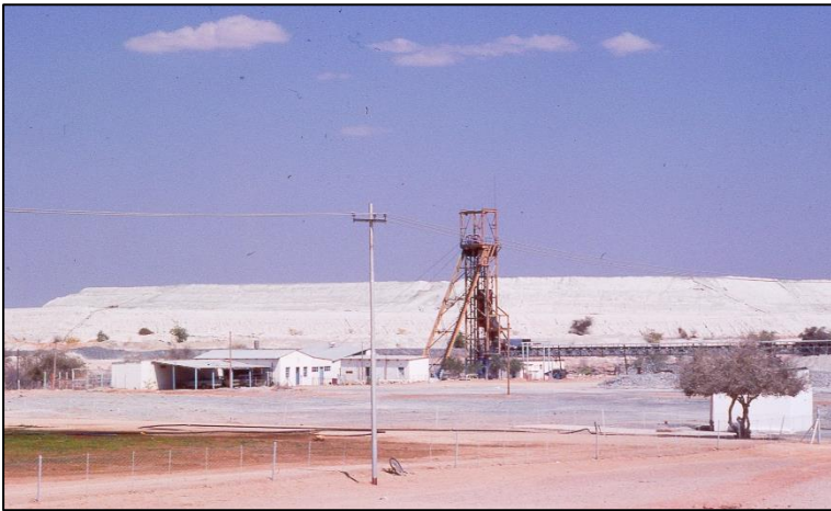
Maria Shaft and tailing dam ca. 1984 (Photo: G Borg)
