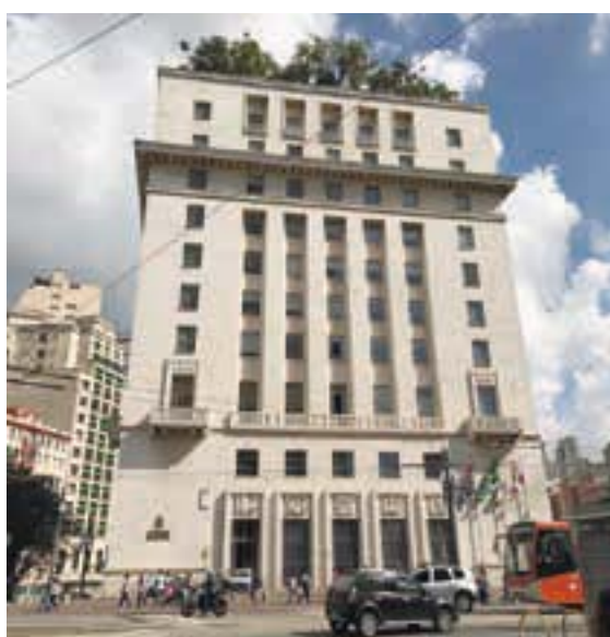
The municipal administration of São Paulo sets a good example of “Urban Greening” with its rooftop garden.
